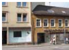
... but some areas face severe development issues.
