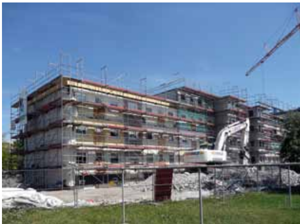
Urban redevelopment in Riesa (Saxony): Reshaping by reducing the number of storeys
