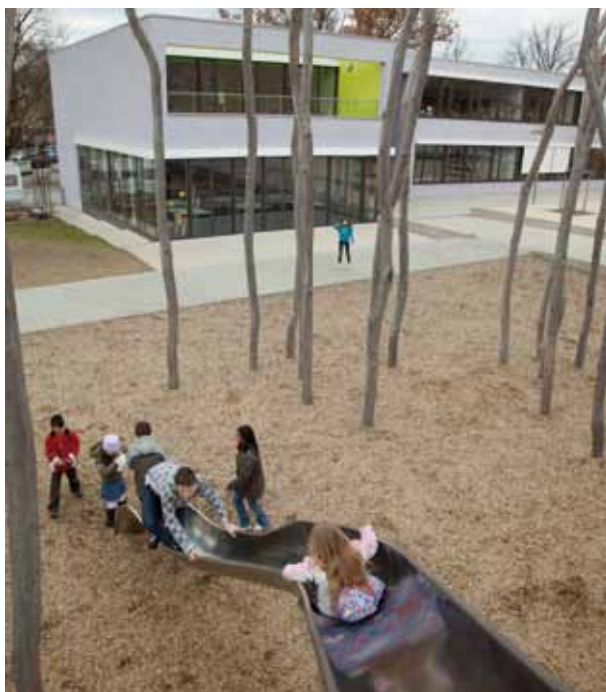
Construction project in Nuremberg district "Nordostbahnhof"
