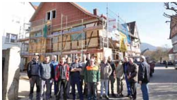
Wanfried Houses project: specimen half-timbered house
