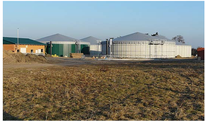
Havelberg in Saxony-Anhalt: the central district heating system was converted into a biogas facility with two block-type heat and power stations. Woodchip heating plants were erected at individual locations, e. g. to supply a Bundeswehr (German Federal Armed Forces) barracks.
