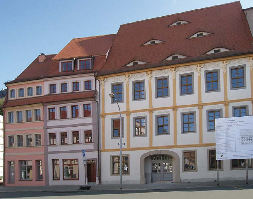
When it comes to energy-efficient retrofit, owners' rights in particular must be taken into consideration. Shown here: these buildings on the market square of the historic centre of Weissenfels have been restored in accordance with heritage conservation and energy-efficiency principles.
