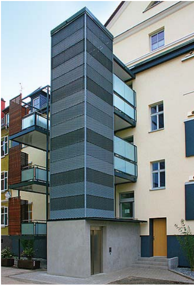
Exterior insulation and new lifts in the courtyard: the historic facades of the Hohenzollern-Höfe facing the street are here to stay.
